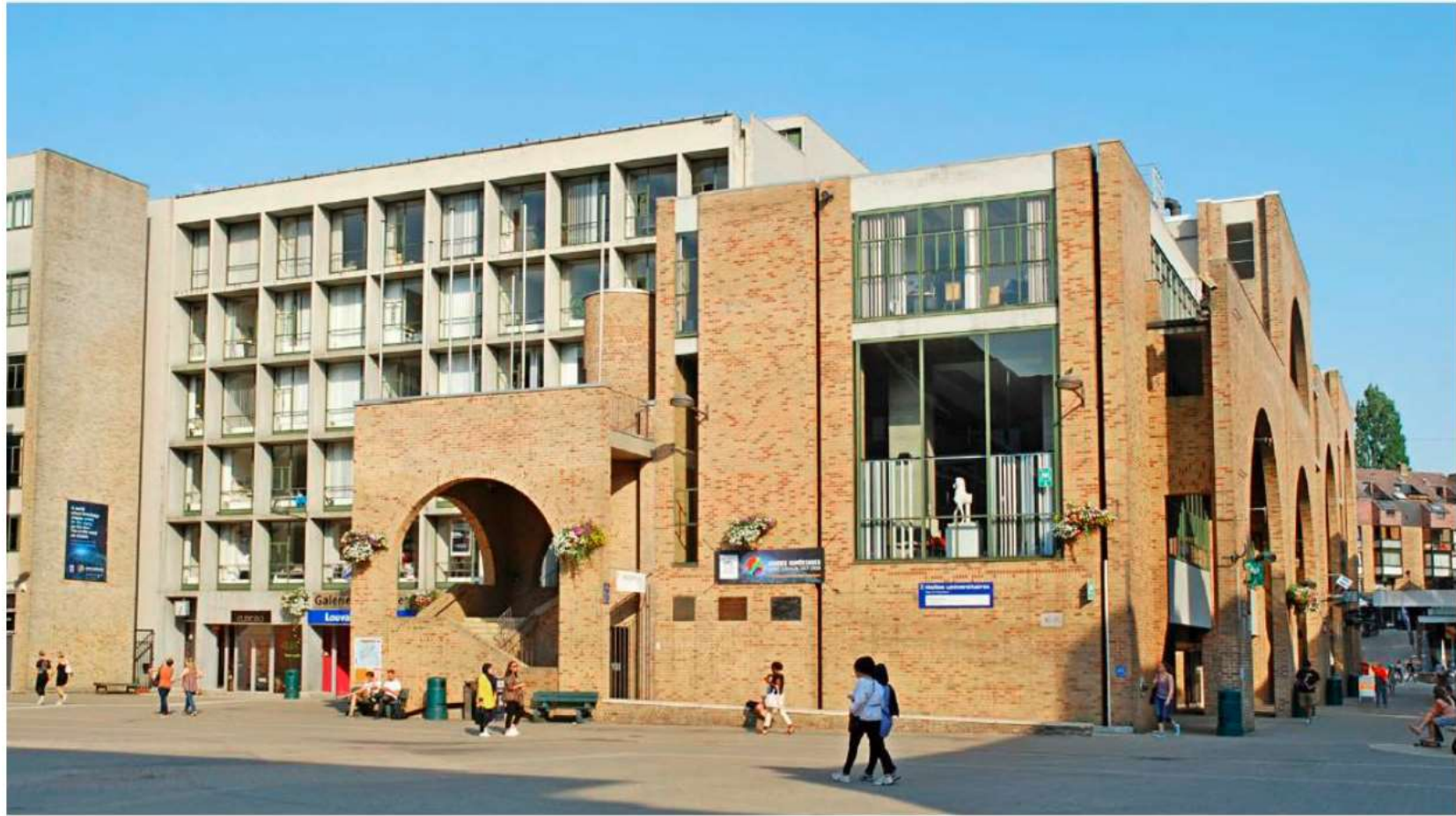
Ill.15. Underground railway station, and university headquarters. Place de l'Université. Photo: Pierre Laconte.
