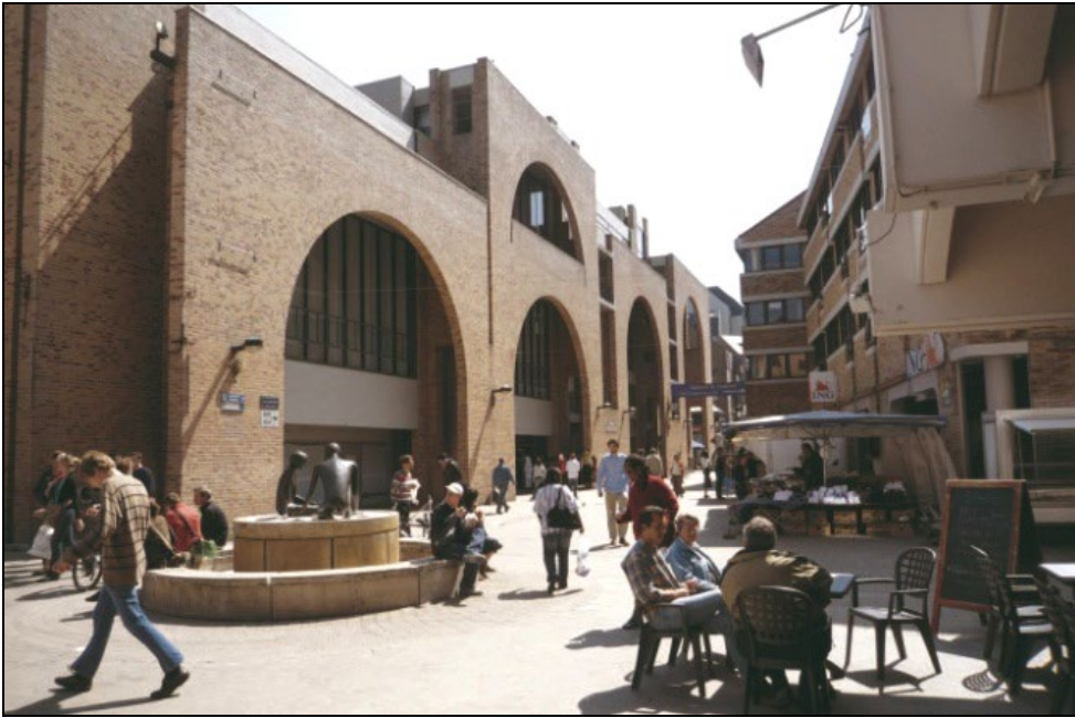
Figure 7.1 - The arcaded entrance to the sub-surface railway station (architect: Y. Lepere) seen from the street level. The station is the point on the pedestrian spine where the natural ground seamlessly meets the artificial ground (i.e. the platform), as shown schematically in Figure 6.
