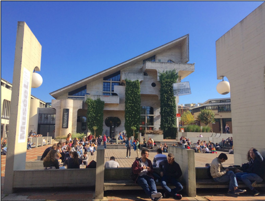
Figure 5.1 - The science library piazza (“Place des Sciences”). This concrete and wood piazza is the main gathering place in the first phase. It includes access to an underpass and to underground parking (photo by Koen Raeymaekers 2018).
