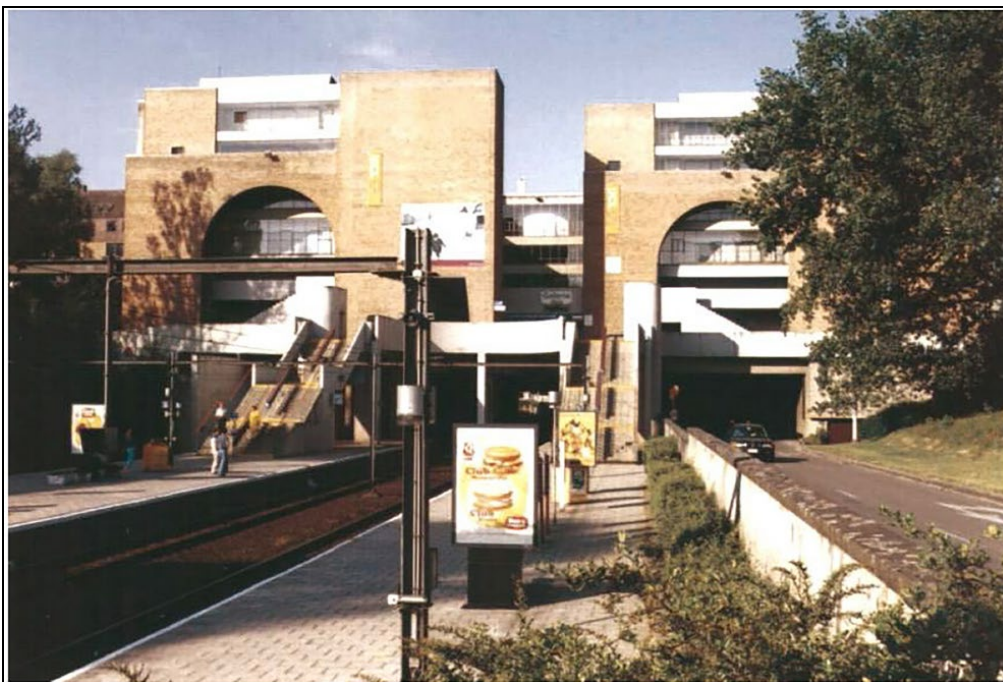
Figure 7.2 – View of the open air tracks, to be expanded. This stations is to become the terminal station of the Brussels Suburban Line 9 and potentially covered.
