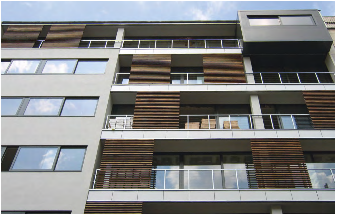
New balconies were built inside the façade. Source : Bureau d'Architectes Emmanuel Bouffieux.
