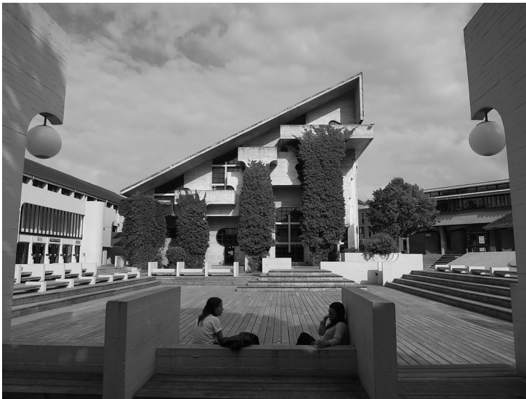
Figure I.1 The Louvain new university town first phase central square, showing the Science Library (architect: A. Jacquemin; overall masterplan and architectural coordination: R. Lemaire, J-P Blondel and P. Laconte).
