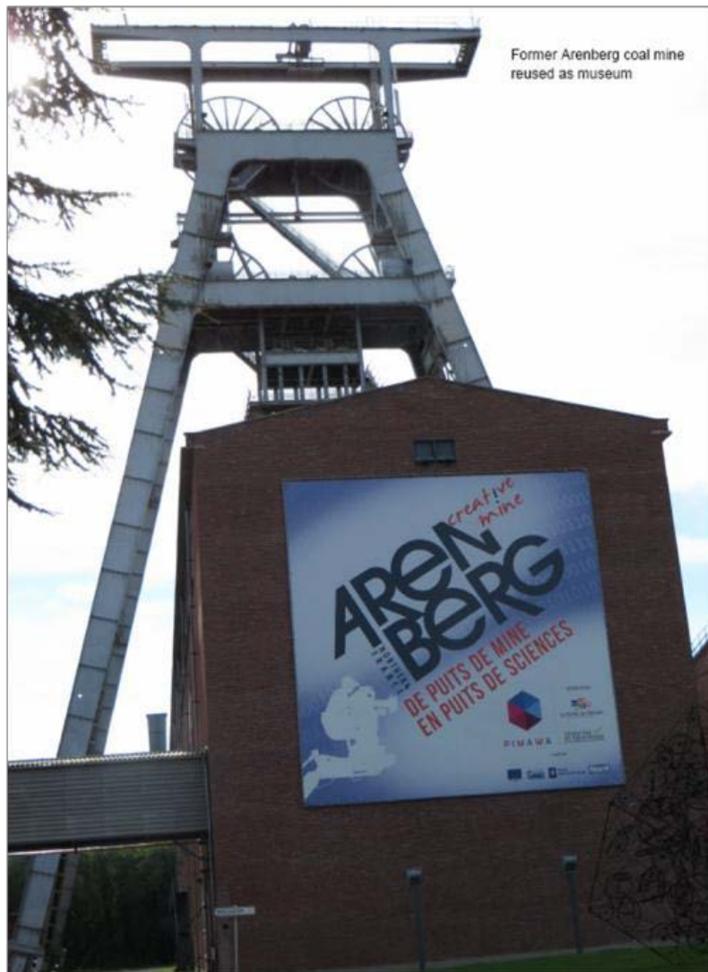
Fig. 6. The Arenberg mining complex, located in the “Bassin minier du Nord-Pas-de- Calais” UNESCO world heritage site, has been restored and is open to visitors. Its visibility has been enhanced through the reuse of part of the site as an engineering university campus publicized as “De puits de mine en puits de science”.
