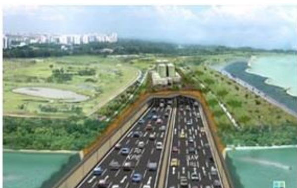
Image 26: Marina Coastal Expressway's 5km long tunnel, Singapore
