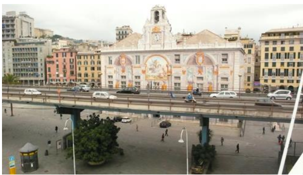
Image 20: the Sopraelevata separating the city center from the ancient harbor
