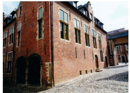
4. View of the entrance to the Beguinage. Credit: André Mertens.
