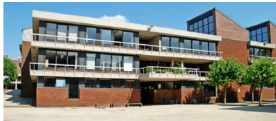
3. Vinci faculty building on the main spine (architect: Gabriel Epstein). Credit: Pierre Laconte.
