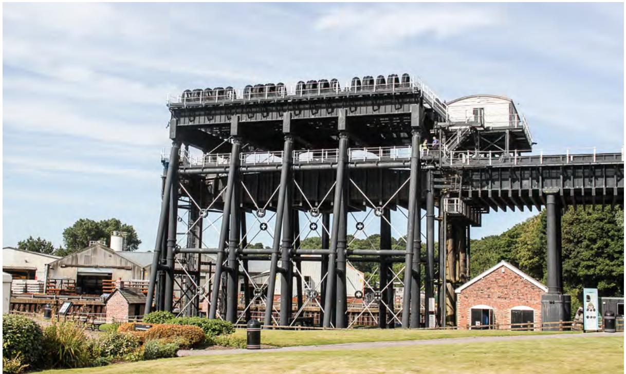
*Below: Near the visitor centre, overhead pulleys and counterweights used for the operation of the boat lift from 1904 until its restoration in 2000*
