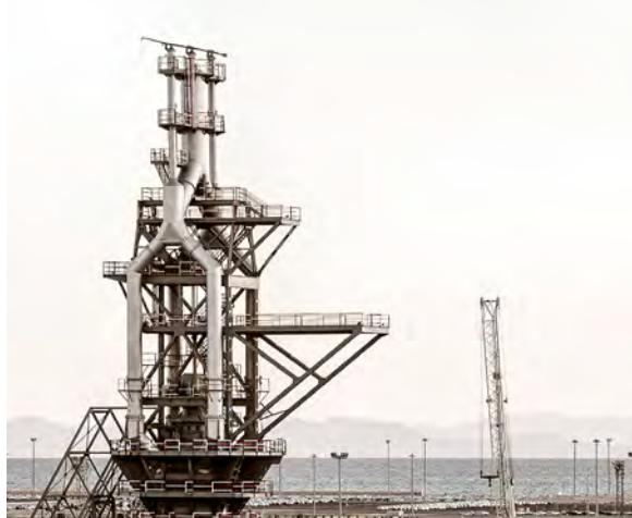
*Piping for furnace gas at the top of the furnace*
