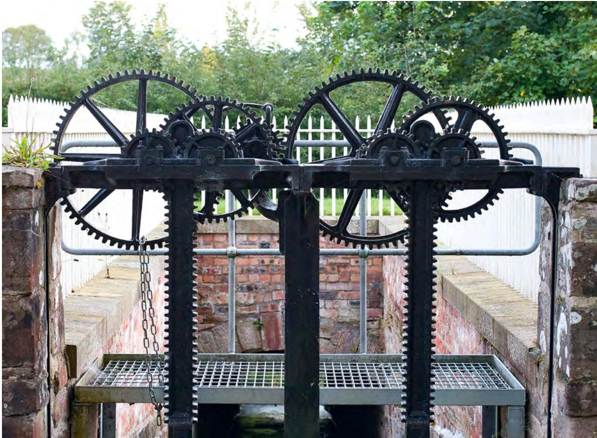
*Above: A sluice gate to control the volume of water going to the wheels. In 1923 a hydro-electric power station came into operation. This takes most of the water today.*
